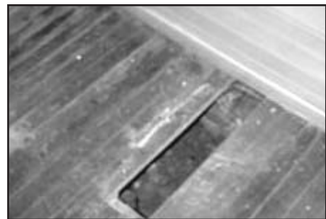
Rotting floor in Efrosini's home.
